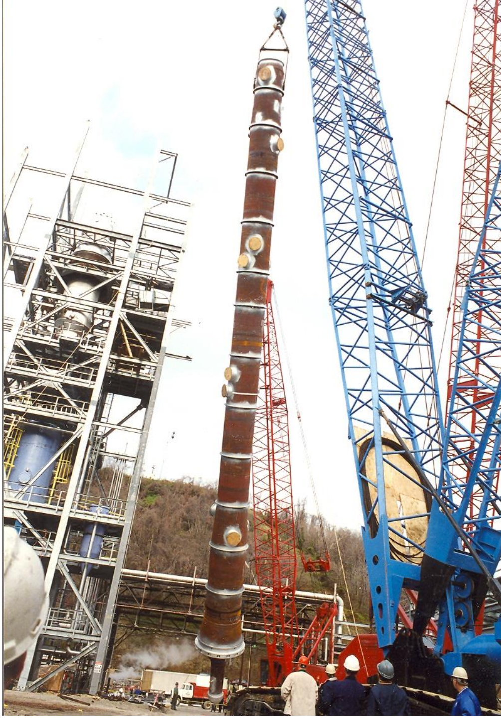
Lampson LTL-350 Transi-Lift 350 ton Lift Crane With 260' boom
